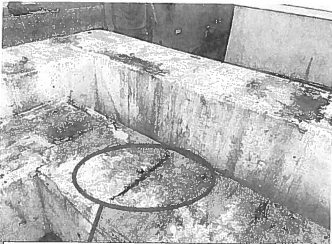
Reseal rooftop air conditioning duct with fab tape and mastic. Rainwater is penetrating the existing ductwork causing leaks inside the building.
